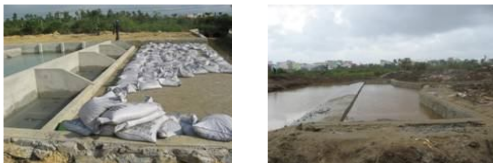
Fig. 2. The settling-filtration tank (left) for controlling run-off water and the overflow dam for controlling water flow to the Sen Lake (right)
