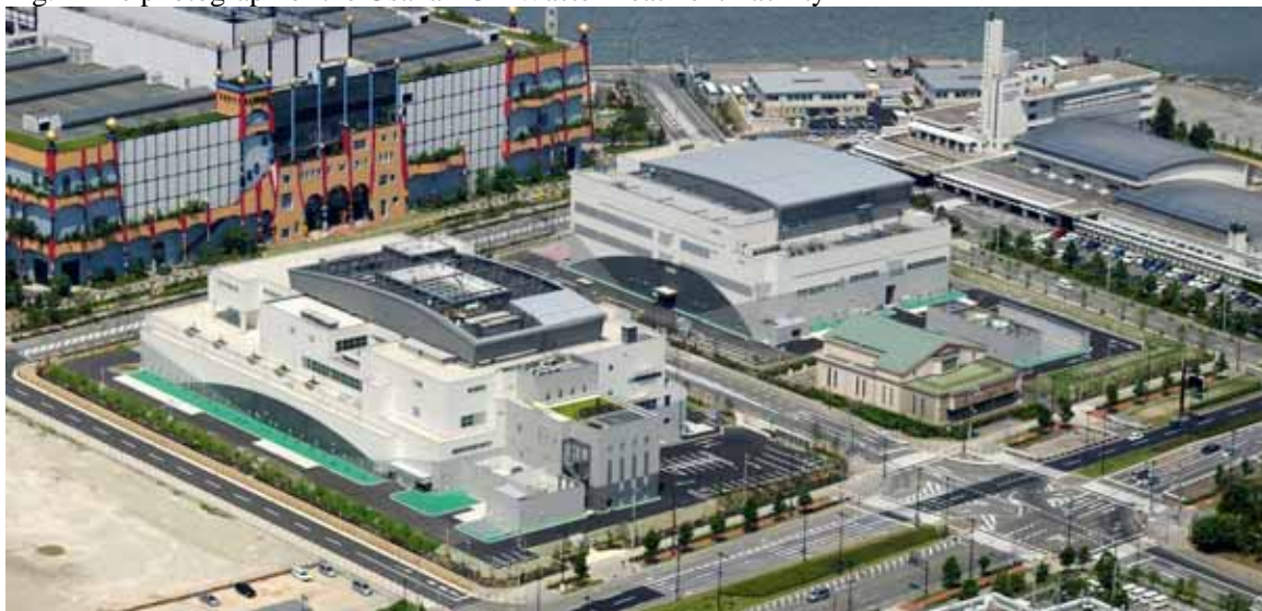
Fig. 1 The photograph of the Osaka PCB Waste Treatment Facility
