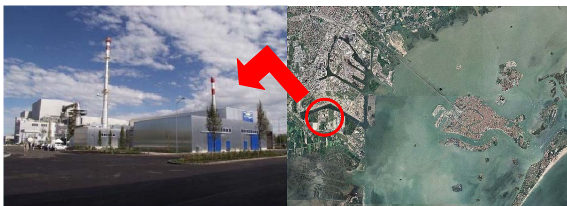
Figure 1: integrated centre of MSW treatment
