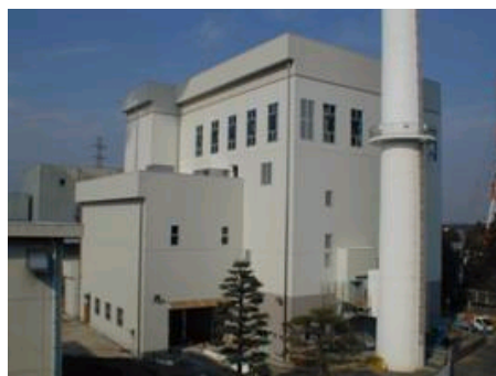
Fig. 3 North Fujisawa Incinerator
