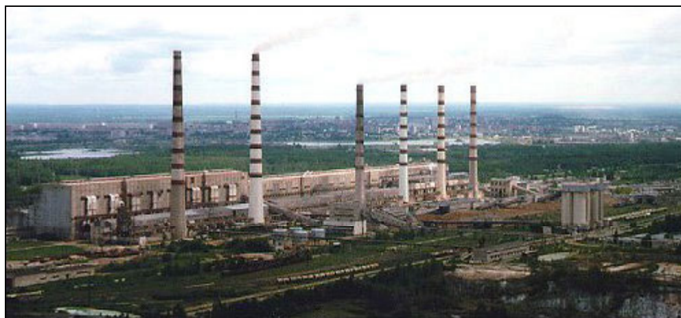
Figure 1. The Balti Power Plant
