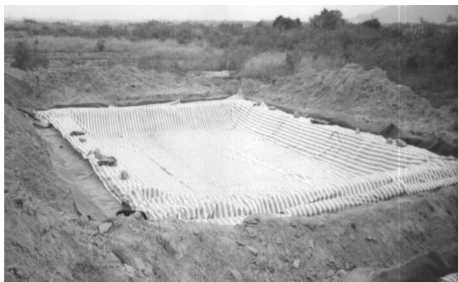
Figure 1. Before “ active landfill ” of toxic chemical contaminated soils in combination with bioremediation treatment at 100 m 3 tria
